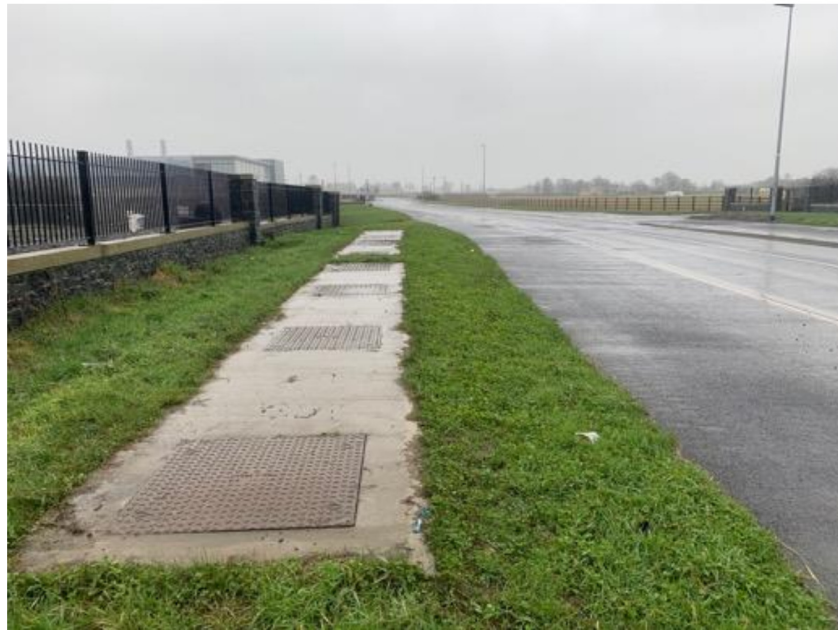
Figure 3 – Baldonnel Rd., south bound
