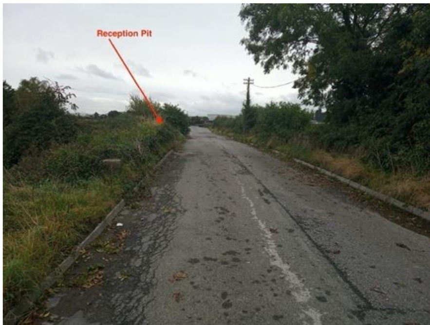
Figure 5 – Reception area on the west site of the Baldonnel Road
